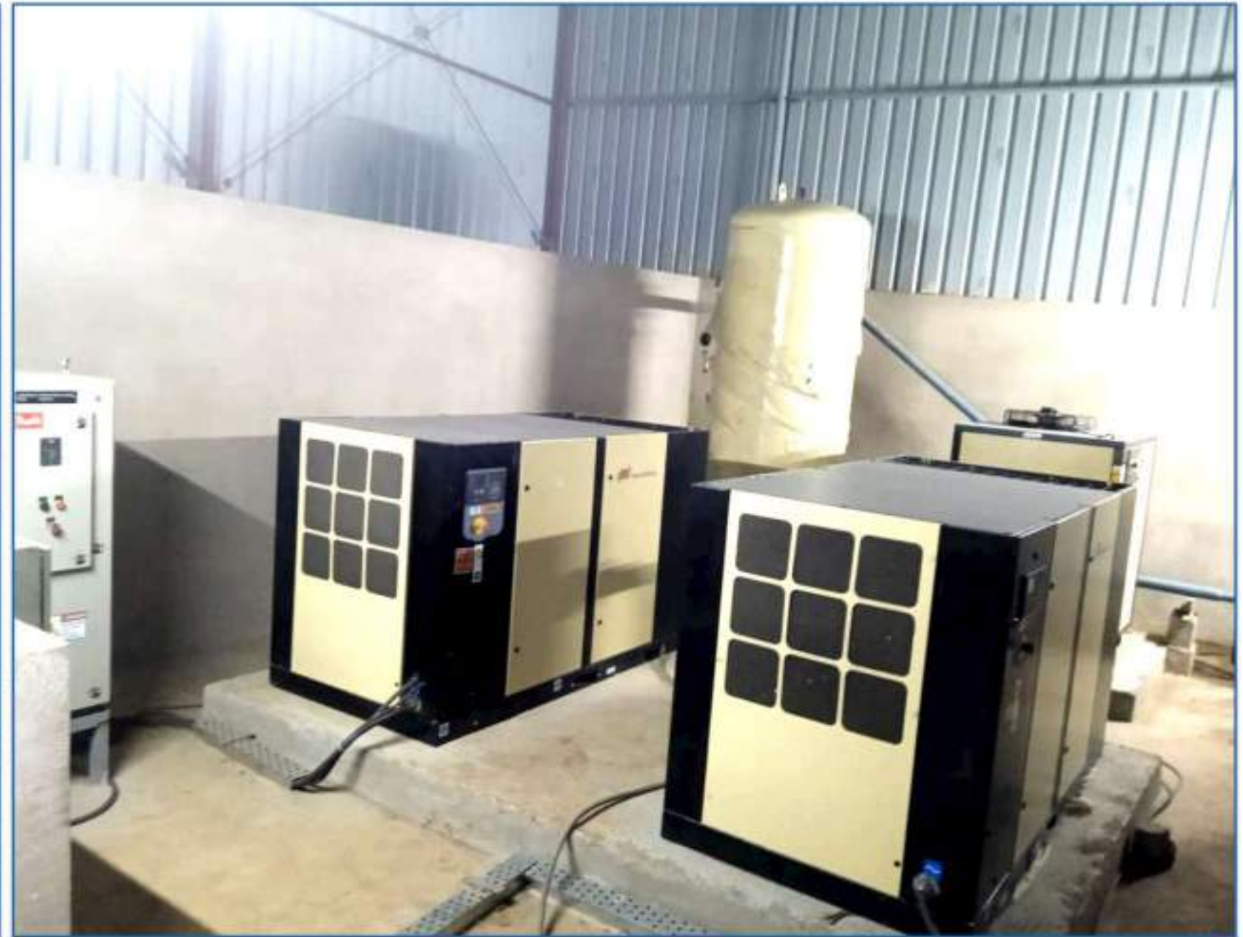
Air Compressor: Air compressors with collective capacity of 600 CFM at delivery of 8 PSI .
